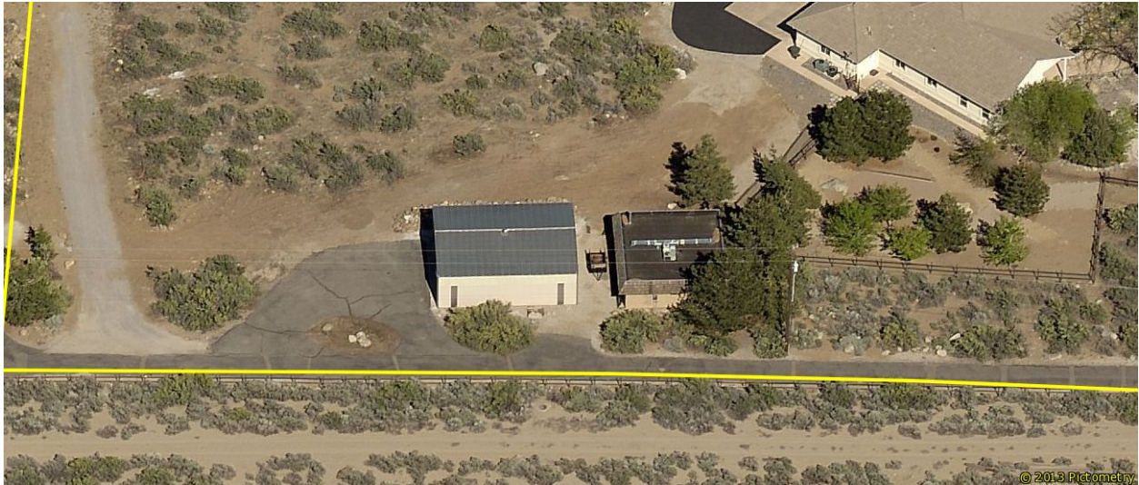
View looking east
